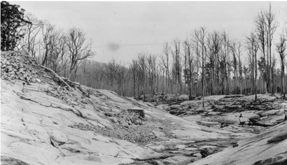
Figure 5. Remains of the Cascade Dam, with ground stripped to bed rock by the flood wave (Source: E. Barsham)
