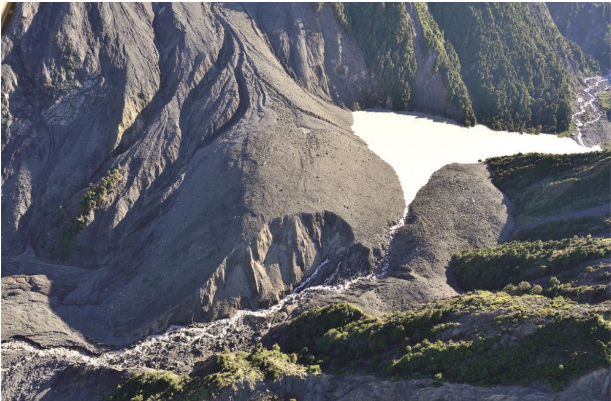
Figure 9. Breach formation from overtopping of the Hapuku River landslide dam, 2017 (Source: GNS Science)
