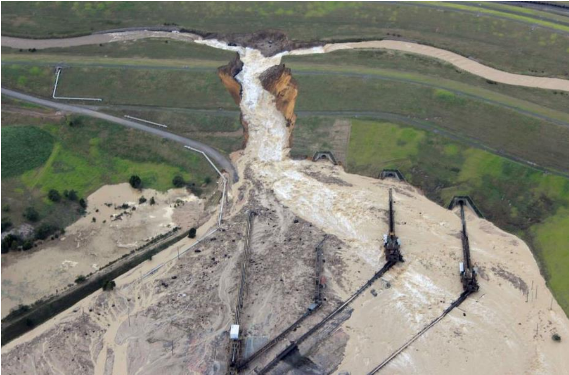
Figure 8. Morwell River Diversion Failure (Source: ABC Network)
