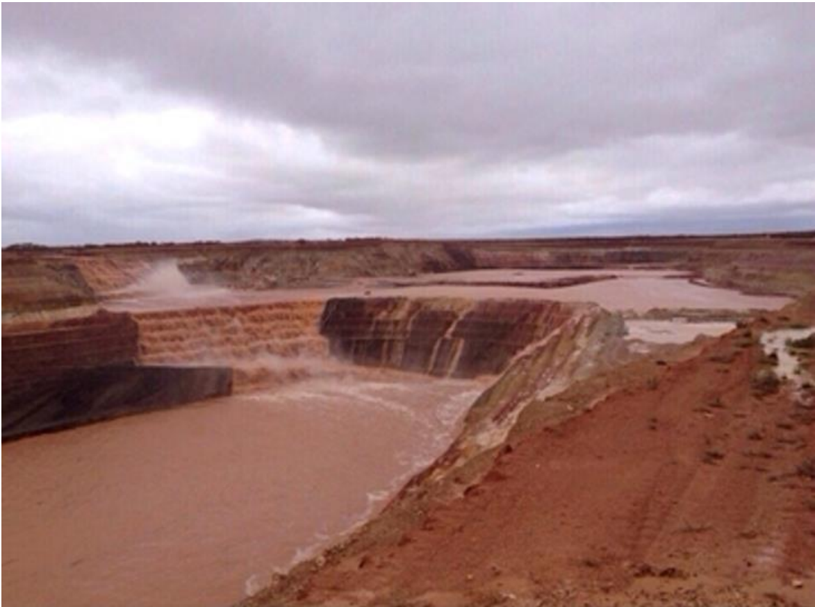
Figure 9. Goldfields pit flooding (Source: Australian Mining)
